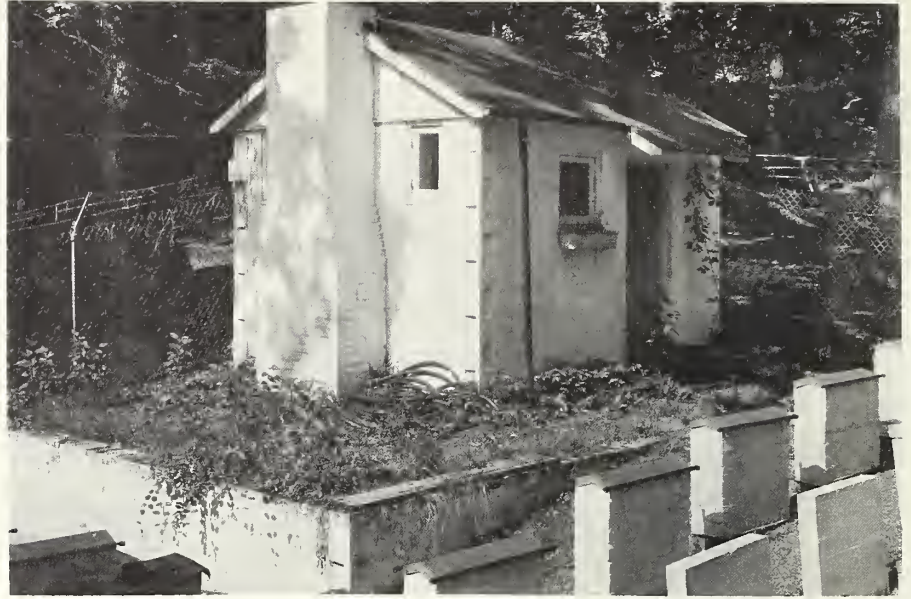
FIGURE 8.3. Cinder-block test house for evaluating durability of coatings for masonry surfaces.
